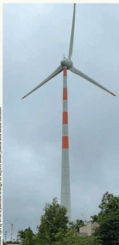
Blade tips of WTG is painted orange to deflect avian fauna and avoid collision
